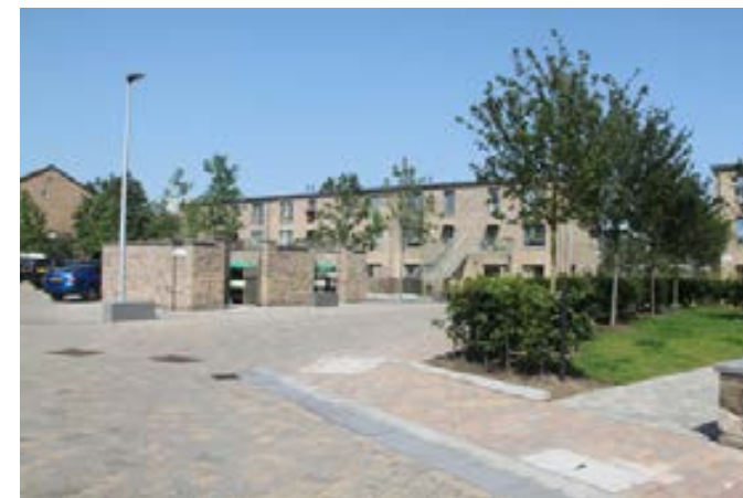
Leith Fort - These carefully designed bin stores are discrete but easily accessible.
