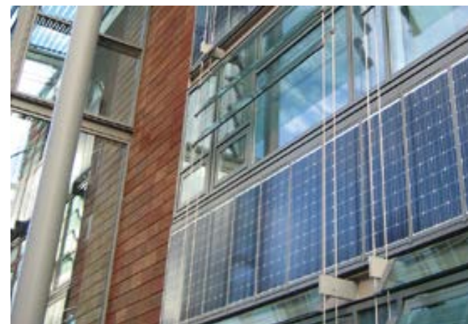
Integrating micro renewables—Kings Buildings Solar Panels are integrated into the design of the elevation.
