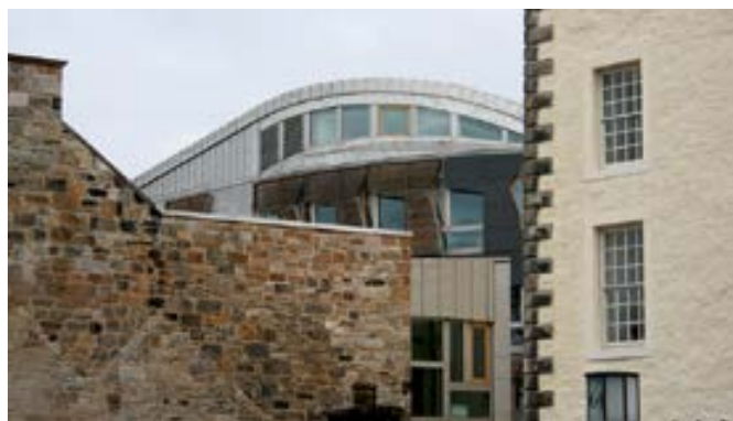
Metal roofing in a historic context — Canongate Stainless Steel roofing has been used on the Scottish Parliament.
