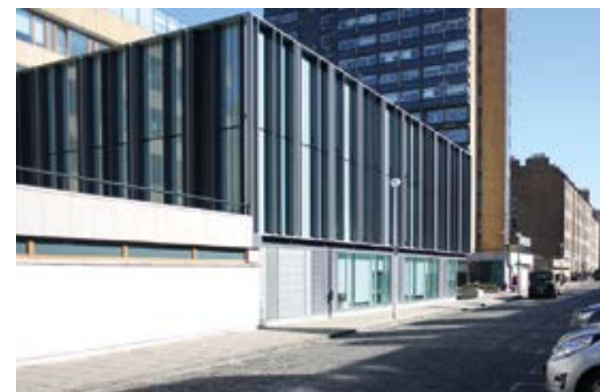
Curtain Walling - Buccleuch Place The potential offered by glazing systems with variations in the window widths, patterning of the glass and mullion depths is fully taken advantage of here.
