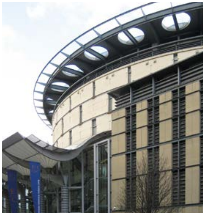
A mixture of cast stone & natural stone—Morrison St. Cast stone was used at high level on the drum shaped part of the building while natural stone was used at low level on the corners.
