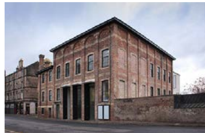
Reusing an existing building—Edinburgh Printmakers Gallery The shell of this building was transformed into a gallery.
