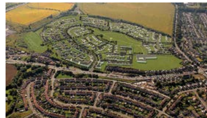
Aerial view of Broomhills Park (Barratt East of Scotland Ltd)
