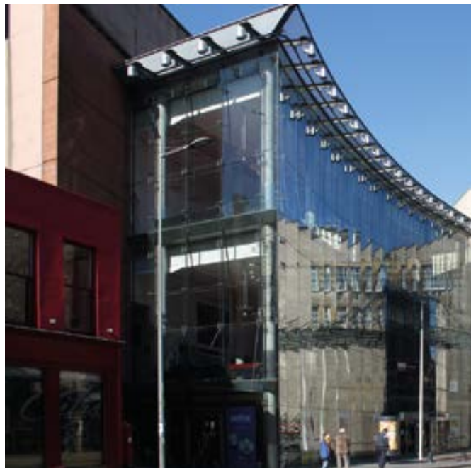
Frameless glazing — Festival Theatre, Nicolson Street The refined detailing of the frameless glazing helps create a striking modern addition to the street.
